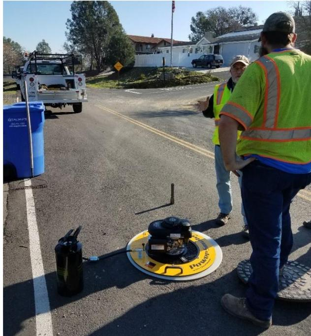
*High-capacity blowers are used to pump smoke into manholes.*
