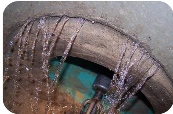
*Inflow such as depicted here can result in an overburdening of the sanitary sewer system, which may result in Sanitary Sewer Overflows (SSOs).*
