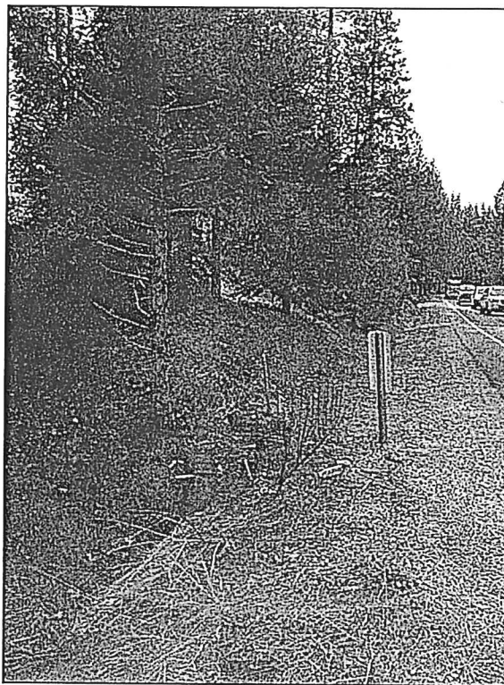
Blue Stake shows existing pipeline alignment at toe of slope
