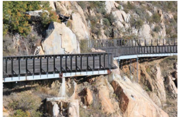
3/4-mile Flume - Utica Power Authority
