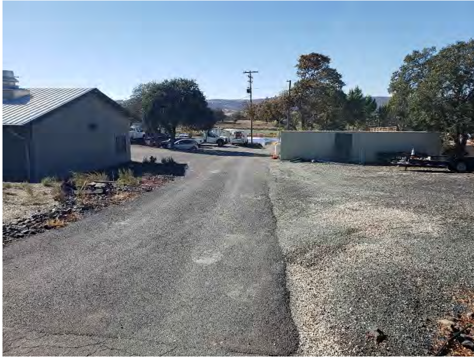
Photograph 5. View of developed area within clearwell portion of the APE, facing West.
