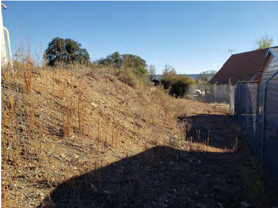
Photograph 7. View of fill used to create the flat surface/platform forming Tank Site B of the APE, facing Southeast.
