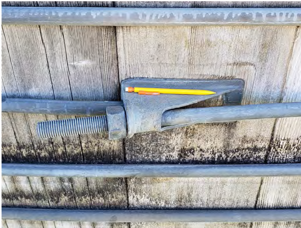
Close-up of metal fasteners which hold redwood tank's metal bands, facing east, taken 11/10/22, Photo #133756, from Photolog BS-01.
