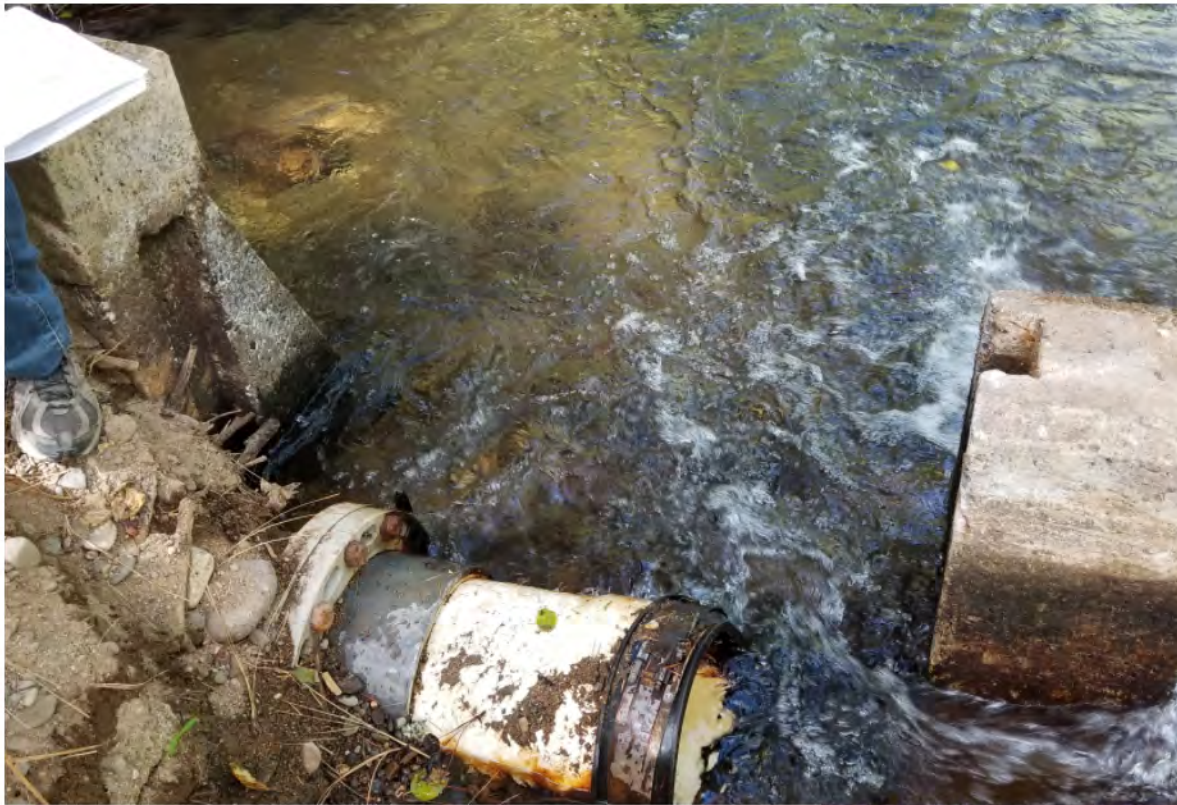
Pump Station Intake Pipe Manifold Removed From Service
