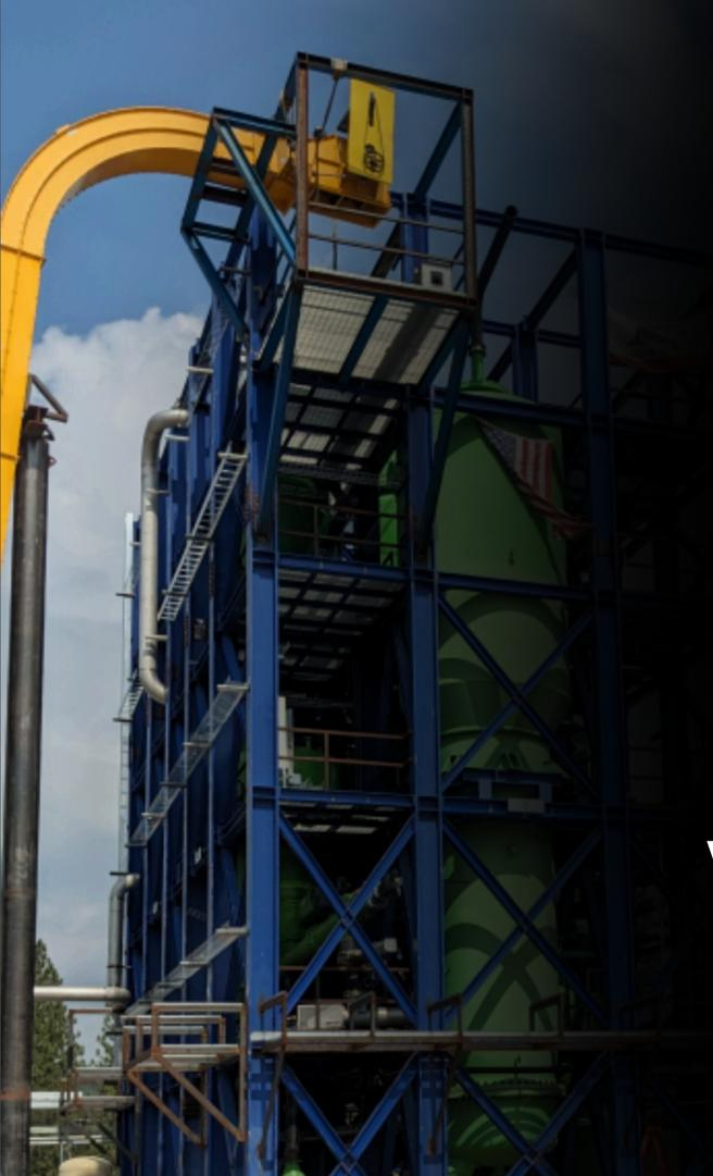
The plant will utilize advanced gasification technology to convert forest waste into clean, hydrogen-rich syngas. Annually, the plant will process around 26,000 tons of logs and chips, reducing the risk of catastrophic wildfire, and improve regional air quality through the reduction of open forest burning.
