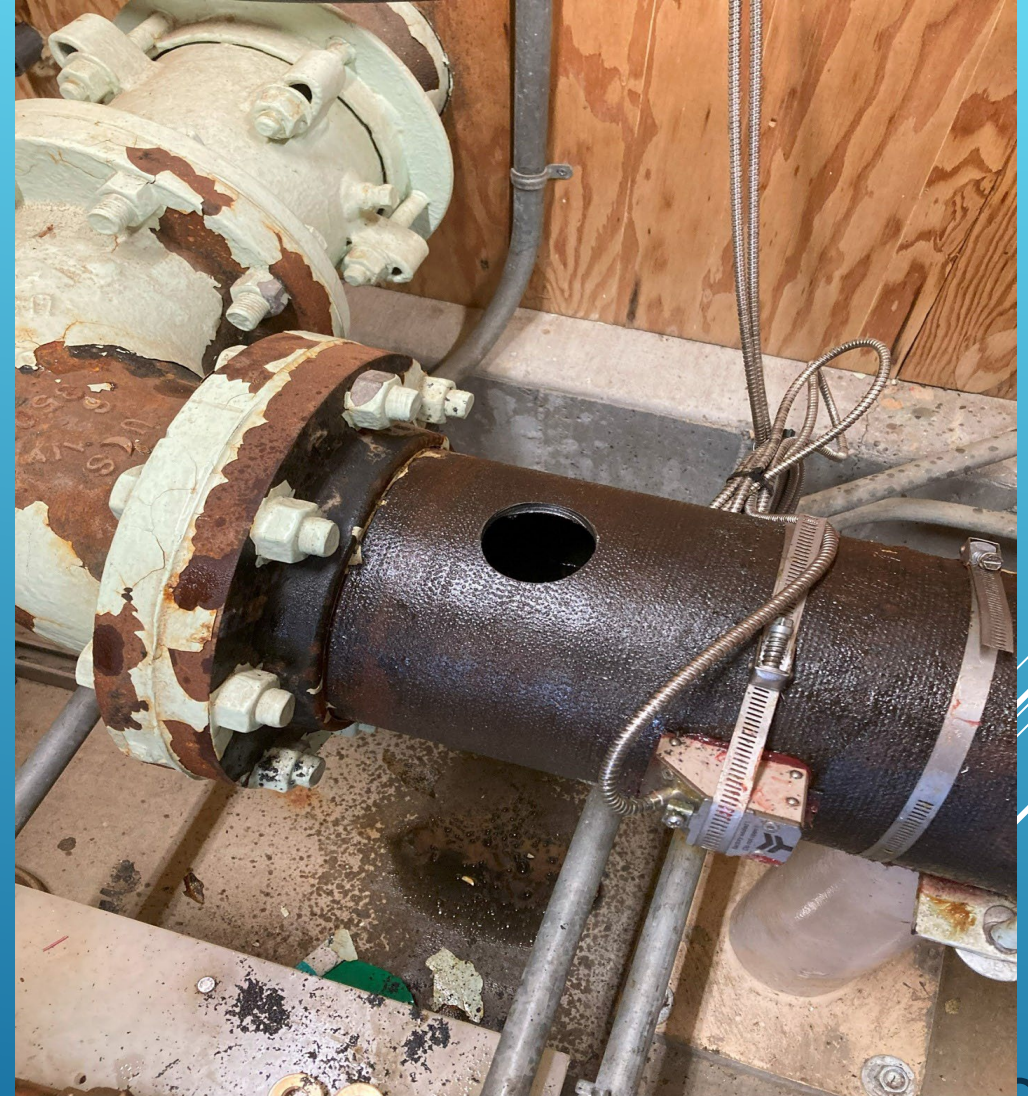
BUOY INSTALLATION – WHITE PINES & TAP OF 6-INCH DUCTILE FOR ARV – FOREST MEADOWS
