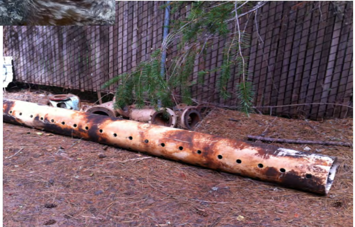
Middle Fork Mokelumne River Pump Station Intake
